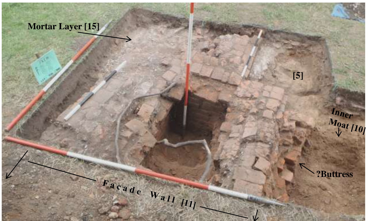
Pl. 2: Inner Moat, Facade Wall, Garderobe Chute and ?Floor Looking East (Photo Neil Pinchbeck)
